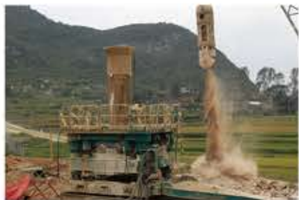
Guiyang Shanghai-Kunming line foundation pile construction
