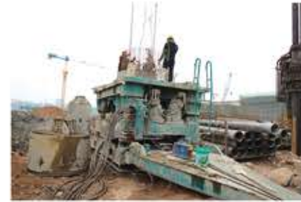
Project construction of Guiyang Guizhou Free Trade Zone
