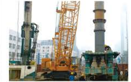
Beijing 14# subway line Pingleyuan Station steel upright post insert construction
