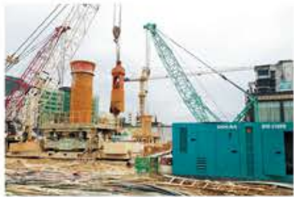
Liuzhou Metro:Secant pile construction
