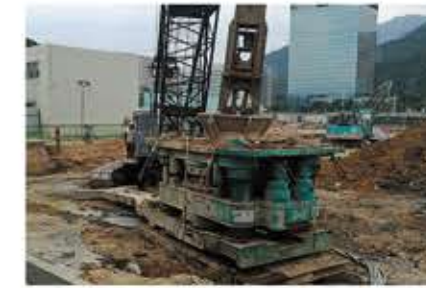
Shenzhen sewage treatment plant project II:secant pile construction
