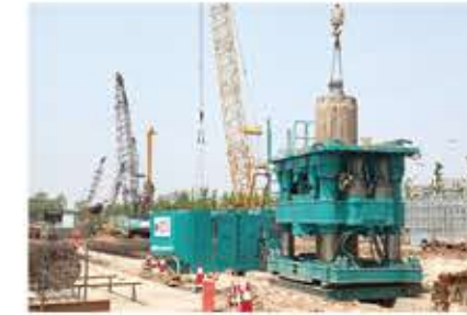
Xuzhou 2# metro line WenBoyuan Station interdigitated pile construction
