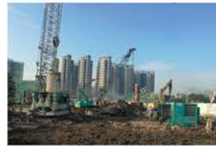
Fuzhou #2 Metro line:Pile pulling construction
