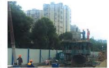
Longyan:China Railway first Bureau XiNan south road Underground passageway
