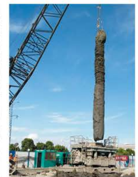
Ningbo rail transit line 4 construction
