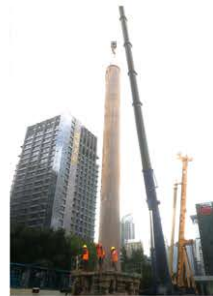
Vanke Shenzhen Binhai landmark project inserted steel column construction
