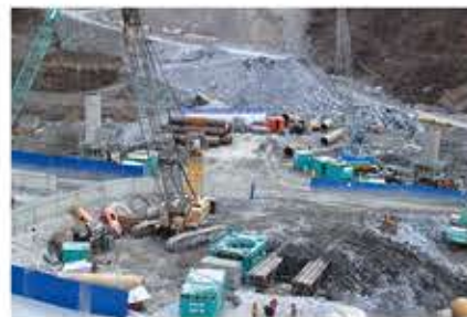
Sichuan Taiping Station of Chenglan railway' s Sixian bridge construction
