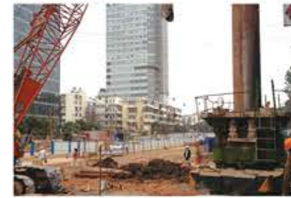
Subway pile foundation construction approaching to Beijing biological bases
