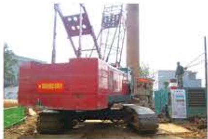
Jiujiang China twenty-four Bureau 's Jiu.Jingqu railway project construction
