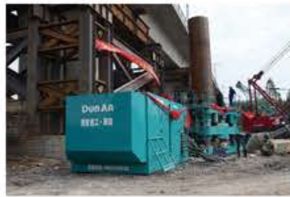
Guiguang high-speed rail construction
