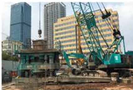
The first people's Hospital of Hefei interdigitated pile construction
