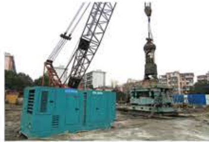
NingBo pile pulling site construction
